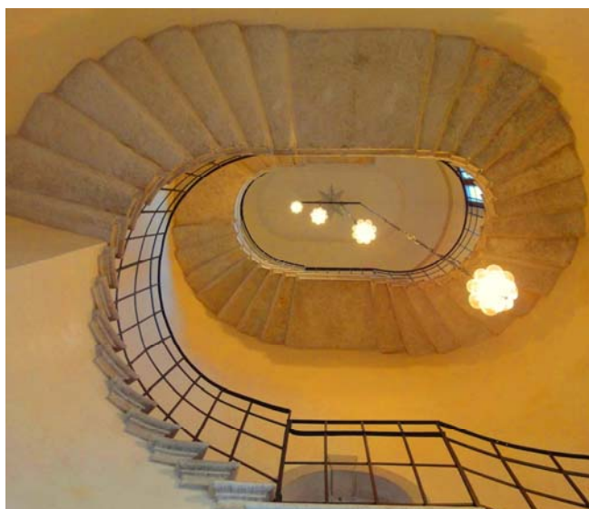
Spiral Staircase, Giorgio Massari arch. (1687-1766) - Cultural Center Don Orione - Artigianelli - Venezia, Italy © Courtesy of the Cultural Center Don Orione - Artigianelli - Venezia, Italy
